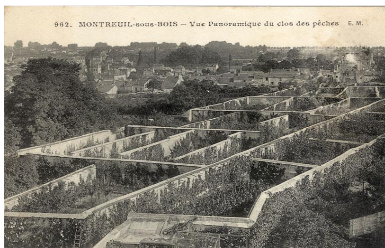
Photo 4. Murs-à-pêches before modernization
